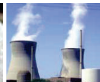
Power & Ash Handling
